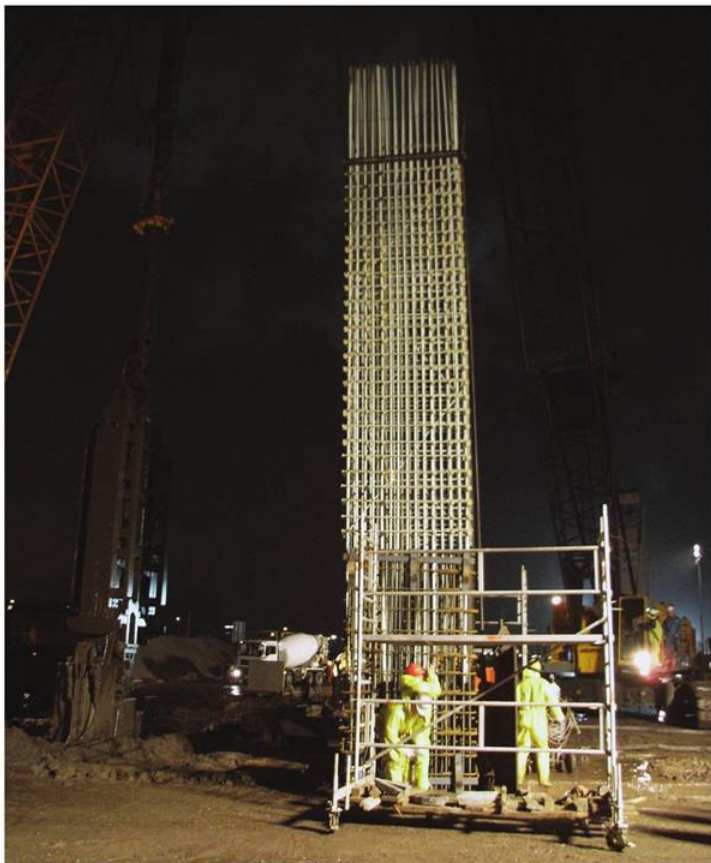
GFRP rebar cage being prepared for installation of the soft-eye.
