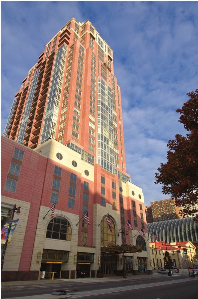
The 31-story Symphony House condominium in Philadelphia used 770 Carbon-Cast Architectural Cladding panels. They weighed 60 percent less than conventional precast, leading to reduced load on the concrete substructure. A smaller building crane was used. HVAC costs are expected to be lower than other exterior wall systems due to superior insulating properties.
