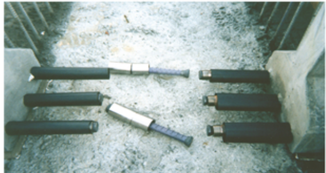
SpliceSeal at San Mateo Bridge job site. Specified by CalTrans (see QPL 09/03). Headed Reinforcement couplers shown.
